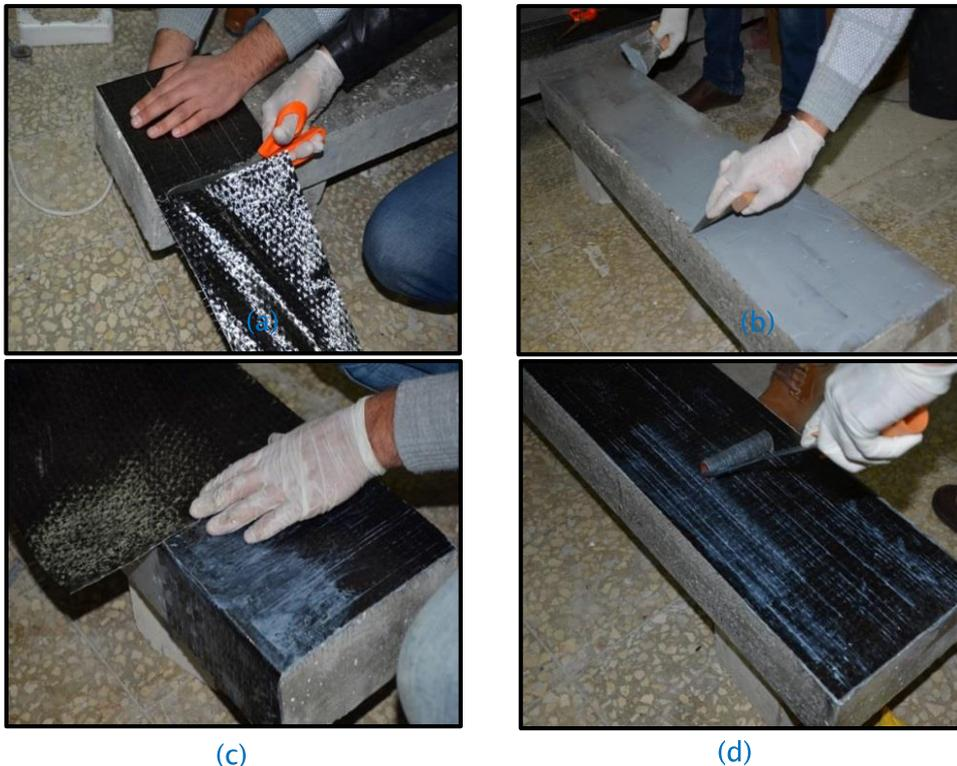
Figure (4): Strengthening process by CFRP sheets: (a) CFRP cutting; (b) Thin layer of epoxy resin; (c) CFRP sheets installation; (d) Remove entrapped air bubbles
