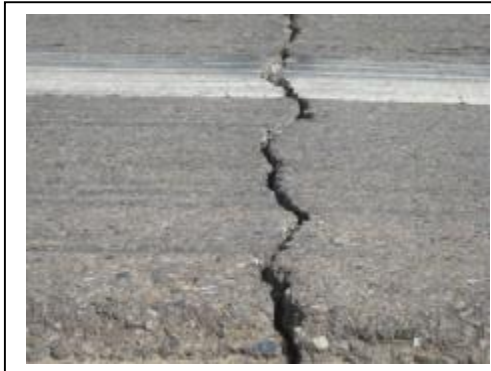
Figure No.B-1 high Transverse Cracking (St. 40+00)
