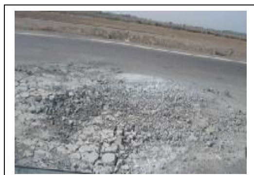
Figure No.B-7 high patches (St. 8+00)
