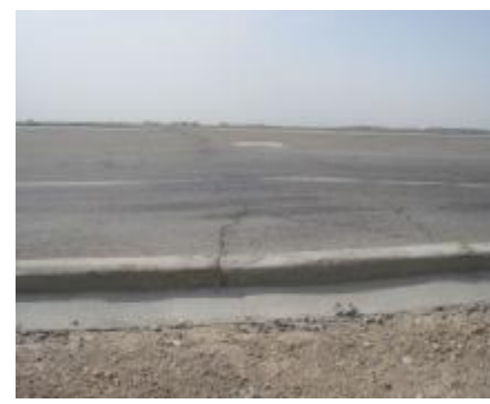
Figure No.B-2 high longitudinal crack (St. 52+00)
