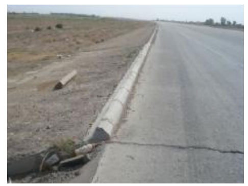
Figure No.B-3 moderate edge crack (St. 30+00)
