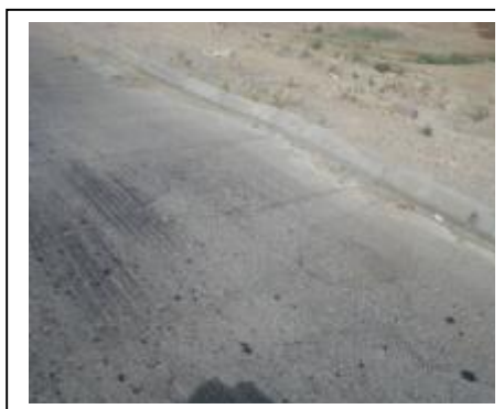
Figure No.B-6 high edge crack (St. 34+00)
