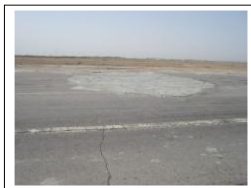
Figure No.B-8 moderate longitude crack and high patches (St. 18+00)
